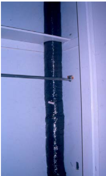
Fig 3-12 Flex insulation over pvc piping
