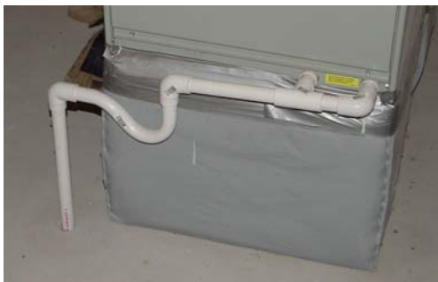
Fig 3-51 Condensation trap
