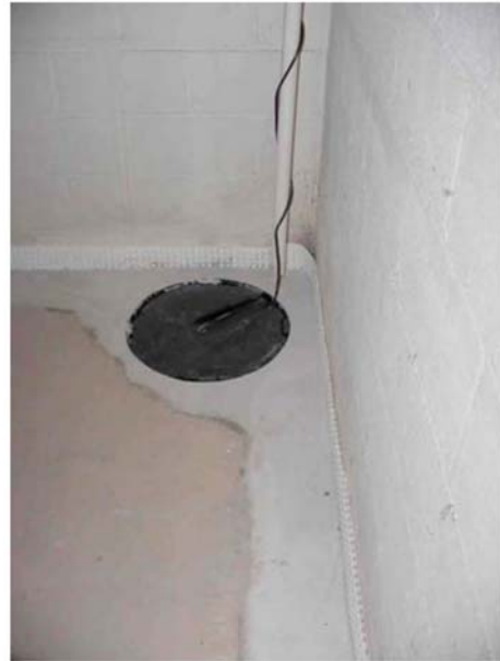
Fig 3-27 De-Watering System
