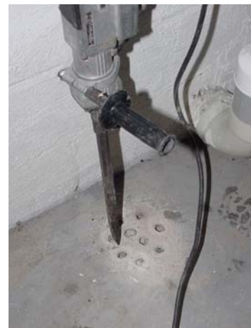
Fig 3-1 Multi-hole Coring
