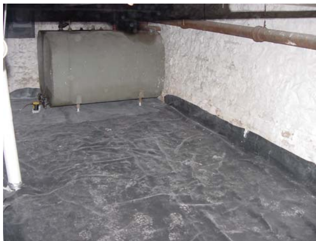
Fig 3-31 EPDM membrane
