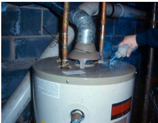
Fig 3-21 Checking draft with smoke
