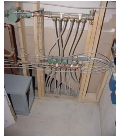
Fig 3-5 Sub-slab vinyl heating pipes
