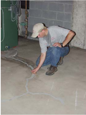
Fig 3-45 Wiping caulk flat
