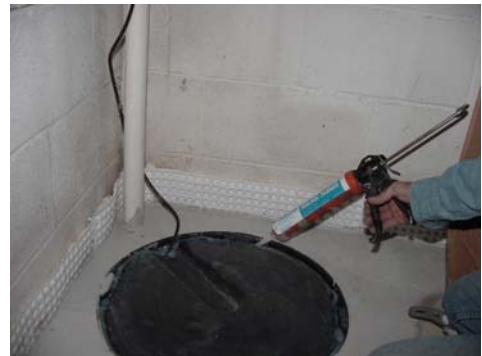
Fig 3-50 Sealing sump cover
