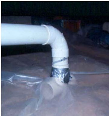
Fig 3-33 CSM dampered suction
