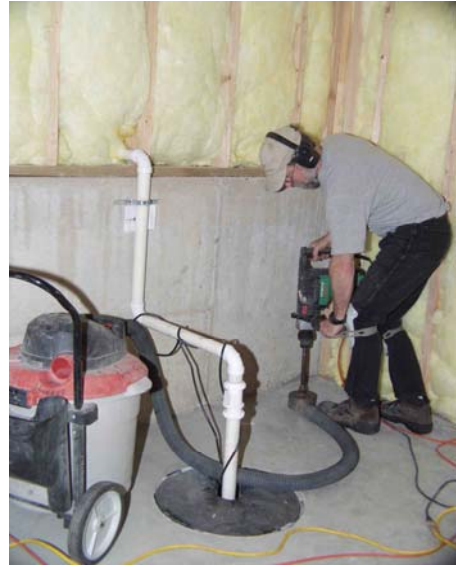
Fig 3-2 Dry Coring
