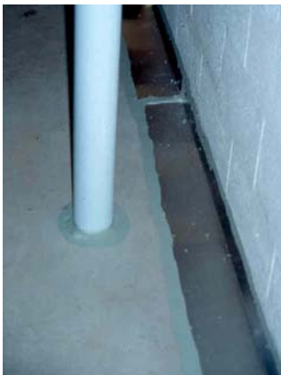
Fig 3-29 Aluminum covering canal drain
