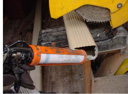
Fig 3-11 Caulking aluminum joints
