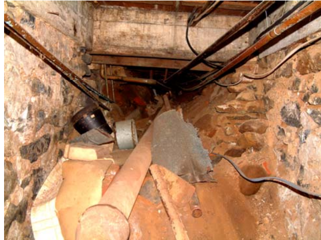
Fig 3-32 Crawl Space debris
