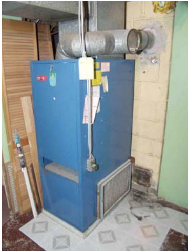
Fig 3-24 No return ducts
