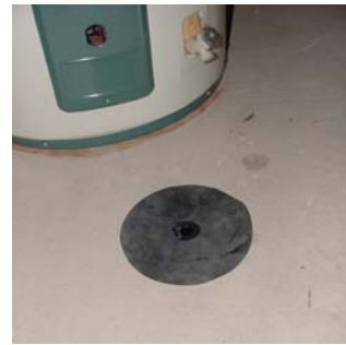
Fig 3-30 one way floor drain
