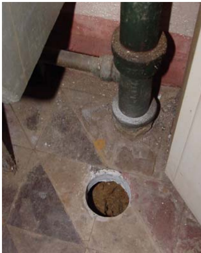
Fig 2-4 Suction Point Near Sub-Slab Plumbing
