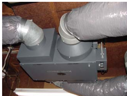
Fig 4-2 Heat Recover Ventilator
