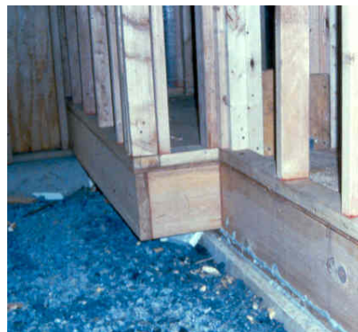
Fig 3-42 Cantilever into a garage
