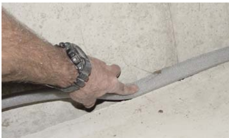
Fig 3-46 Installing backer rod
