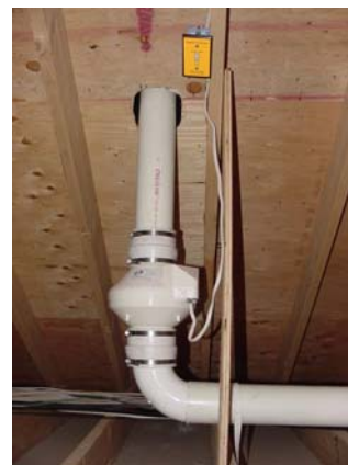
Fig 3-7 Fan in attic
