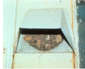
Fig 4-3 Blocked HRV intake
