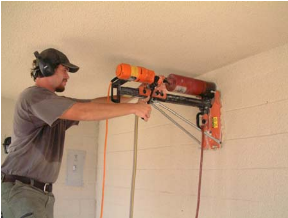
Fig 3-3 Wet Coring
