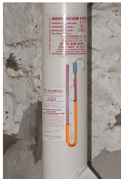
Fig 3-16 u-tube manometer
