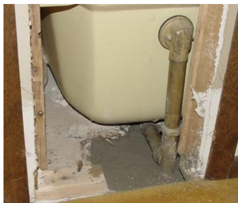
Fig 3-47 Sealing under a tub
